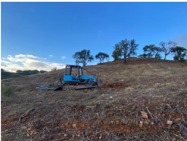
Clearing the land
